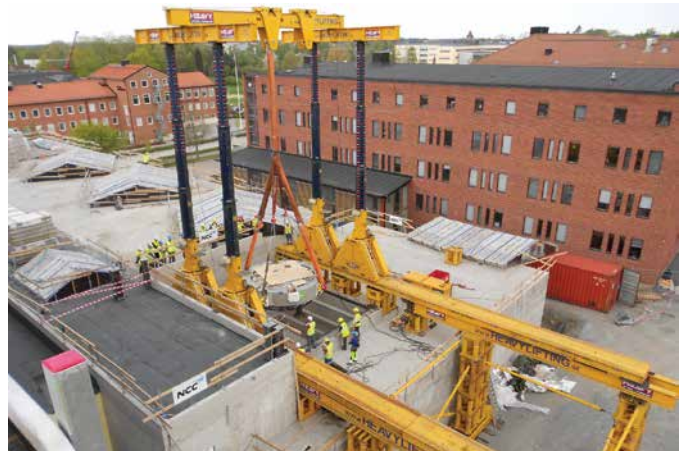
Figure 10 – Cyclotron lift at Skandionkliniken PBT facility in Sweden (source: http://www.cranestodaymagazine.com/news/heavy-lifting-install-cyclotron-in-sweden-290513/ ).
