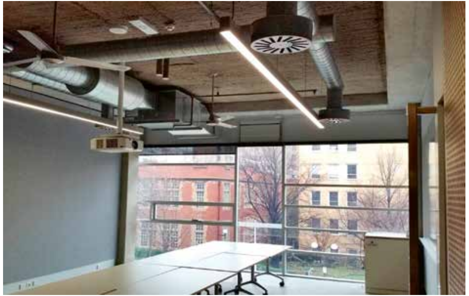
Mixed-mode ventilation was a challenge for the design team.
